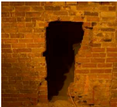
I4: Brick Load Bearing Wall Alteration. Monastery of the Visitation of Holy Mary. Jason. Carleton University. 11-04-2019
