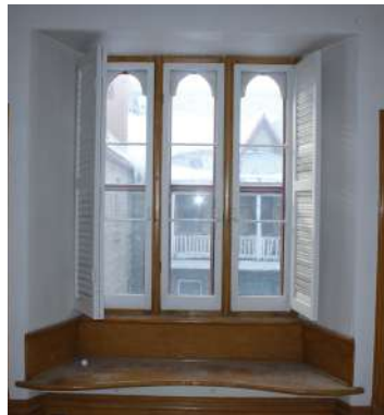
E27: Wooden windows in good condition. Monastery of the Visitation of Holy Mary. Jason. Carleton University. 11-04-2019
