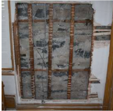
I2: Lath and Plaster Removed. Monastery of the Visitation of Holy Mary. Jason. Carleton University. 11-04-2019
