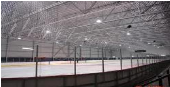
Trusses in arena
