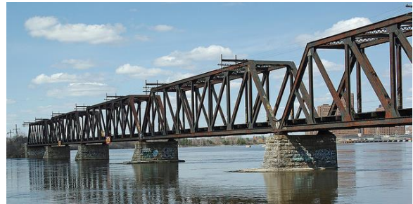
Over-Truss steel bridge
