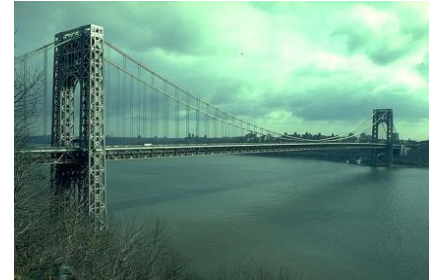
Cable supporting bridge
