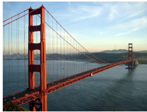
Golden Gate Bridge
