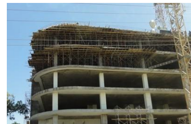
Reinforced concrete slabs
