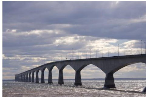
Confederation Bridge - Canada
