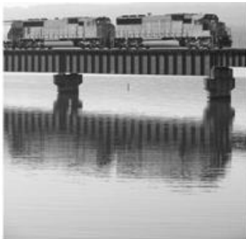
Figure: FG06_02UN Design of this bridge girder is based on influence lines that must be considered for this train loading.
