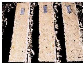
16-yr old concrete (Type 50, w/c = 0.39)
