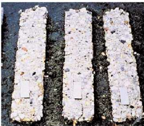
12-yr old concrete (Type 50, w/c = 0.65)
