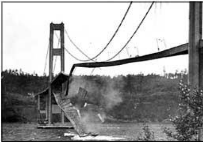
TACOMA NARROWS SUSPENSION BRIDGE COLLAPSE, 1940
