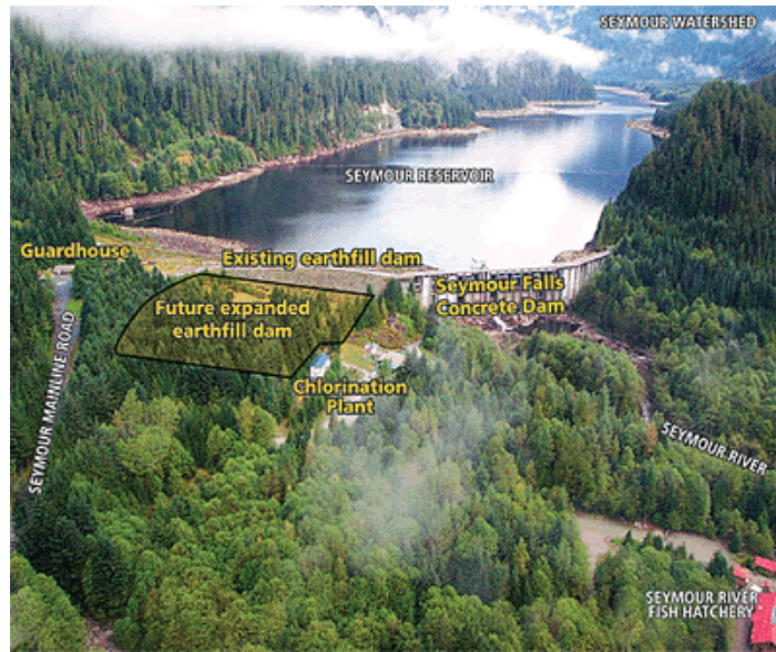
Figure EQ.61 Seymour Falls and the planned upgrades projected for completion by 2007. The upgrades will ensure that the Dam performs safely in the event of a major earthquake. Photo from Metro Vancouver.
