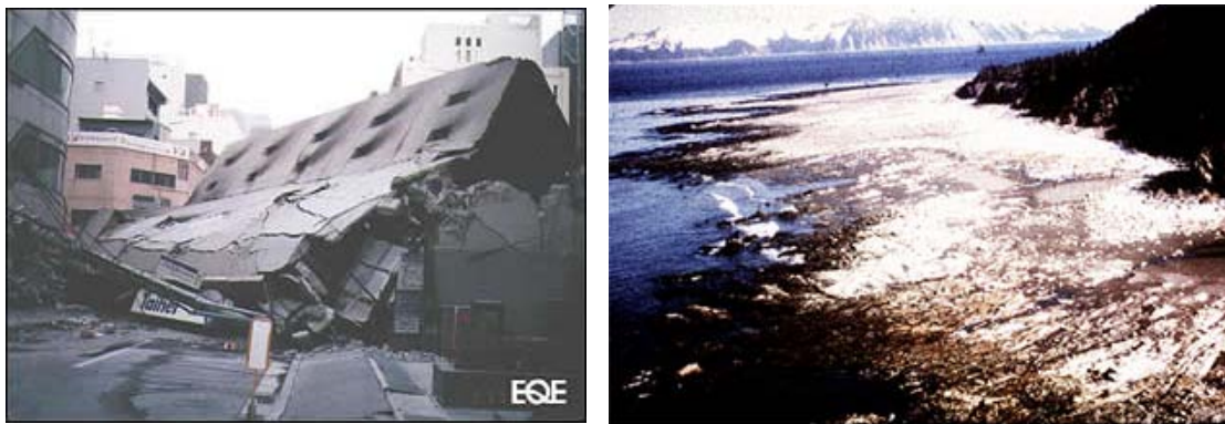
Figure EQ.53 The figure on the left shows some of the damage and destruction in Kobe, Japan after the earthquake in 1995, M_w=7.2 . The damage to infrastructure was estimated to be $2.7 billion and cost 6,425 lives. The figure on the right shows an intertidal platform that was uplifted 33 feet during the 1964 Good Friday earthquake in Prince William Sound, Alaska, M_w=9.2 . The damage caused by the earthquake was estimated to be between $300-400 million but only cost 116 lives in Alaska. Basic information on these and other earthquakes may be found at the USGS website.
