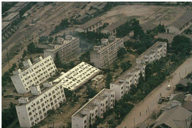
Figure EQ.66 (Left panel) Photo of buildings that were destroyed because of liquefaction following an earthquake near Niigata, Japan, 1964. (Right panel) Photo of an earth dam that was very nearly breached (water breaking through) as a result of liquefaction caused by earthquake shaking. Less than a minute more of shaking and the
