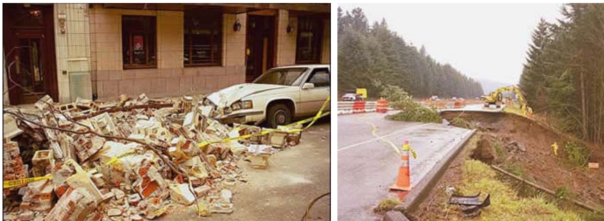
Figure EQ.11 Images of damage to buildings and cars near the Washington Capitol Building in Olympia, WA (left) and to Highway 101 (right). Photos retrieved from The Nisqually Earthquake Information Clearinghouse.
