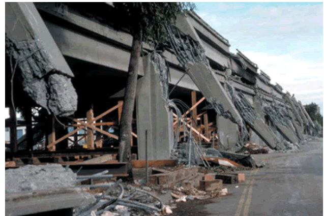
Figure EQ.65 (Top left panel) An entire city block in Kobe, Japan burns following the 1995 M_w 6.9 earthquake. Photo from City of Kobe, Japan (Top right panel) Map showing areas devastated by fire, Kobe, Japan, 1995. (Bottom right panel) Side view of support-column failure and collapsed upper deck, Cypress viaduct, Oakland, California. Photo credit: H.G. Wilshire, U.S. Geological Survey.
