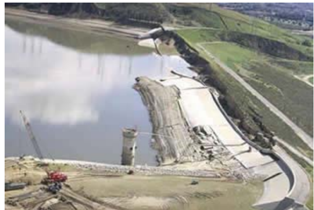
Figure EQ.66 (Left panel) Photo of buildings that were destroyed because of liquefaction following an earthquake near Niigata, Japan, 1964. (Right panel) Photo of an earth dam that was very nearly breached (water breaking through) as a result of liquefaction caused by earthquake shaking. Less than a minute more of shaking and the
