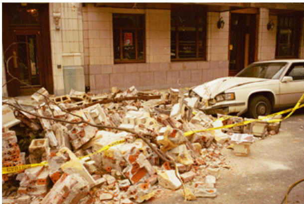
Figure EQ.64 (Top left panel) Bricks that fell because they were not properly attached to a building near the Washington Capitol Building in Olympia, WA causing damage to cars and other properties on the ground. Photo retrieved from the U.S. Geological Survey and The Nisqually Earthquake Information Clearing House (Top right panel) Concrete failure at the joint between two sections of reinforcing, Interstate 880 in California.
