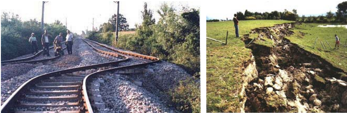
Figure EQ.16 (Left panel) A displaced a railway line caused by a strike-slip fault rupture following the earthquake in Izmit, Turkey, on August 17, 1999. (Right panel) Rupture caused by movement on the Fault near the city of Bam, Iran.
